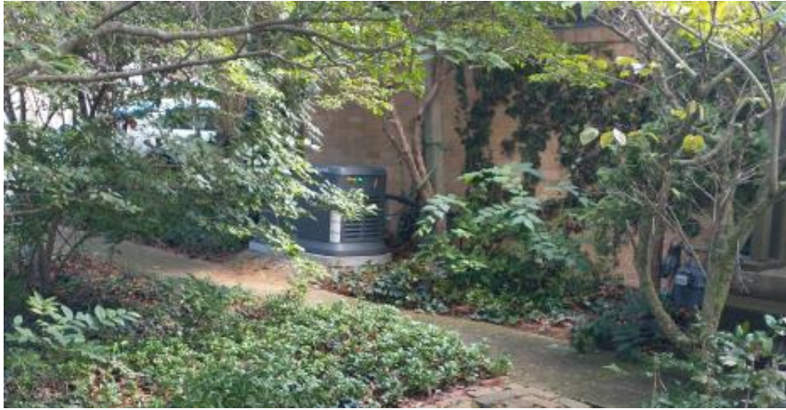
view of equipment in front yard – east of driveway
