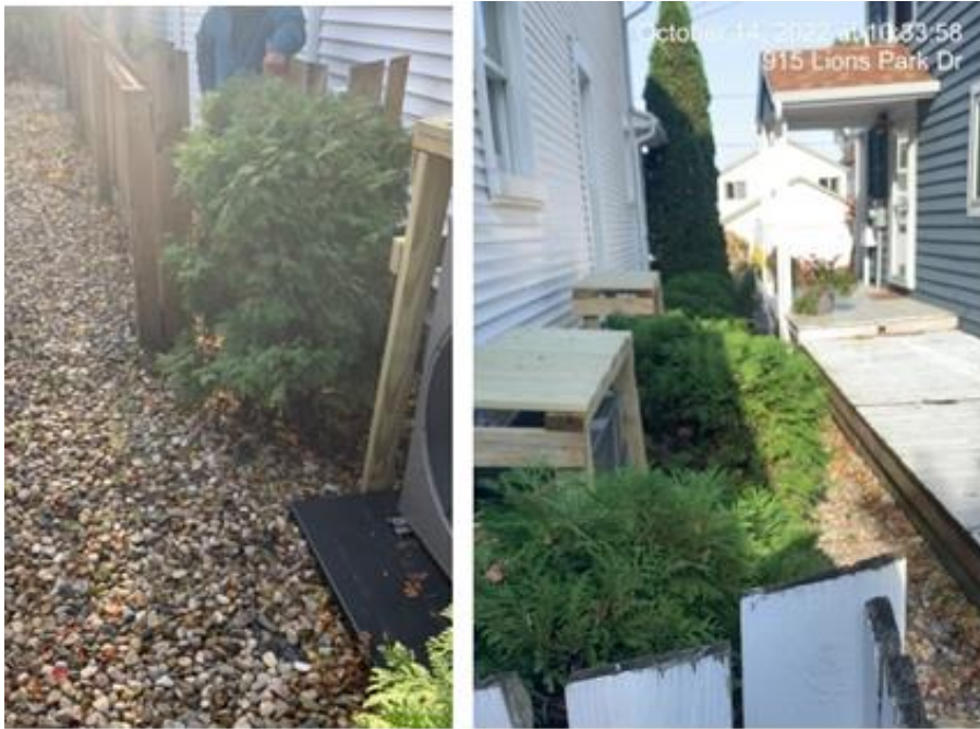
2 units relocated 9-18-24 photo
