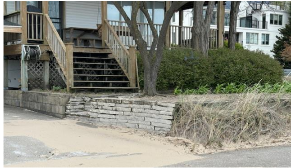
Limestone retaining wall
