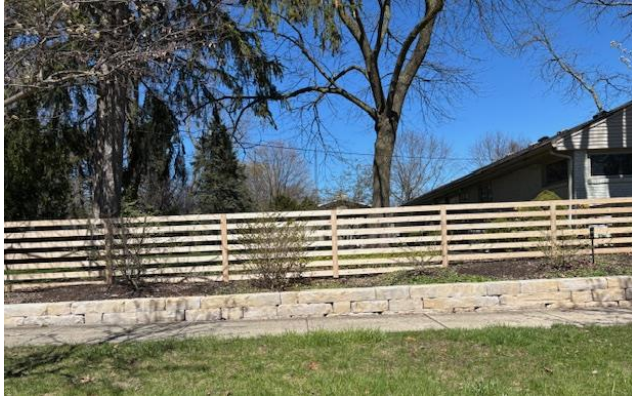
Landscape block retaining wall with fence
