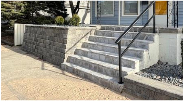
51" tall Garden wall same level as front porch
