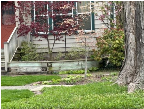
Garden wall adjacent to dwelling
