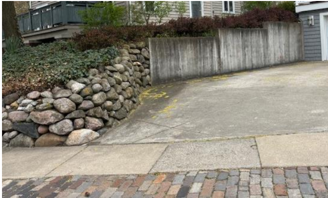
Rock and concrete retaining wall
