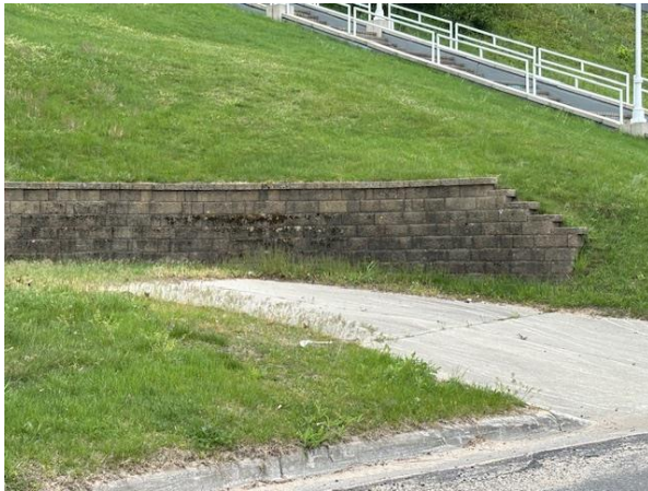
Landscape block retaining wall
