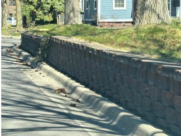
Landscape block retaining wall
