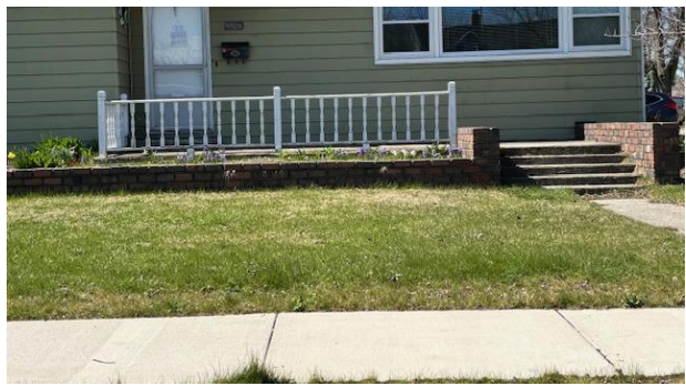
Garden wall with fencing at entrance
