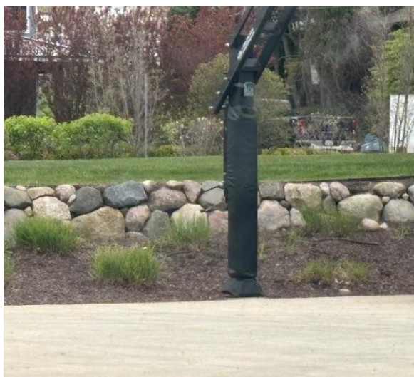
Rock retaining wall
