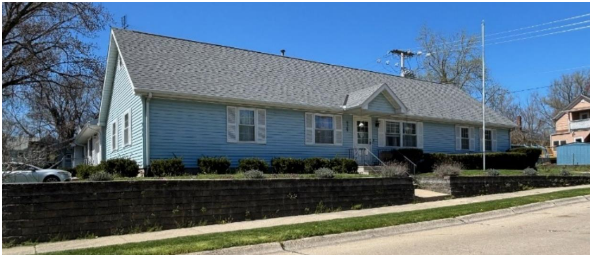
Landscape block retaining wall
