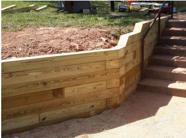
Wood timber retaining wall
