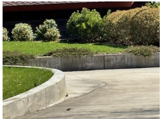
Concrete retaining wall
