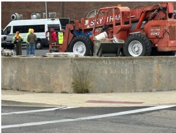
Concrete retaining wall
