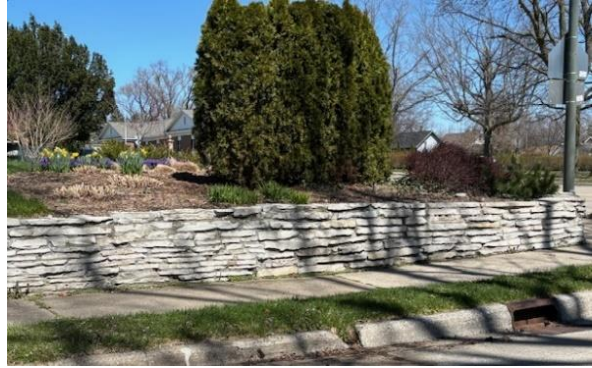
Limestone retaining wall
