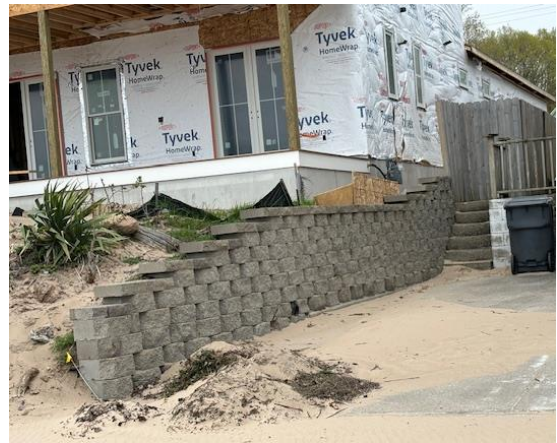
Landscape block retaining wall
