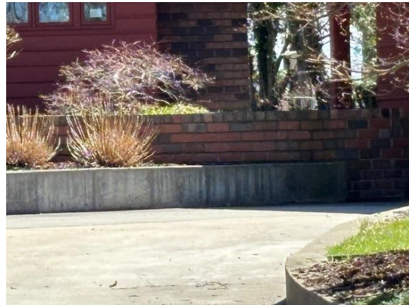
Concrete and possibly brick retaining wall
