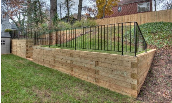
Wood timber retaining wall with fence
