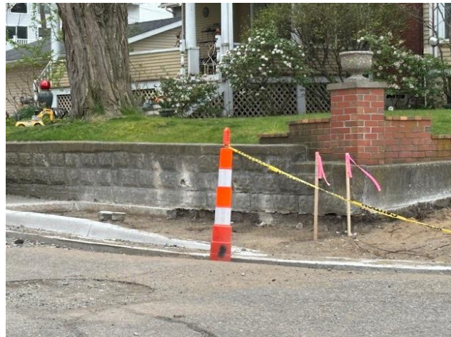
Landscape block and concrete retaining walls
