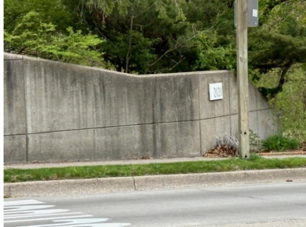
Concrete retaining wall
