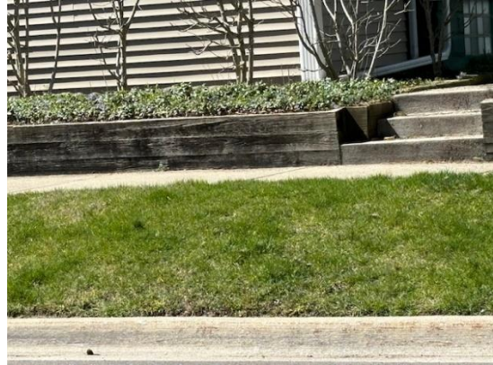
Wood timber retaining wall
