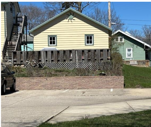
Brick retaining wall with fencing
