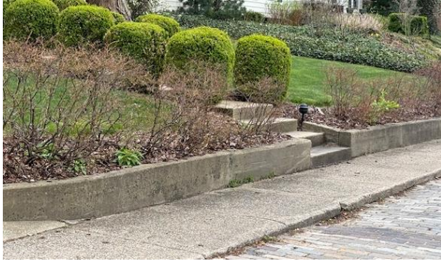
Concrete retaining wall
