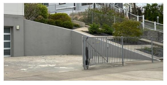
Concrete retaining wall with front yard fence
