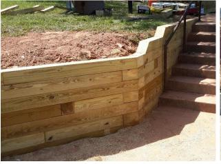
Wood timber retaining wall
